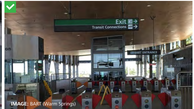
IMAGE: BART (Warm Springs) Permanent signs hung judiciously from ceiling, preserving sightlines and architecture.
