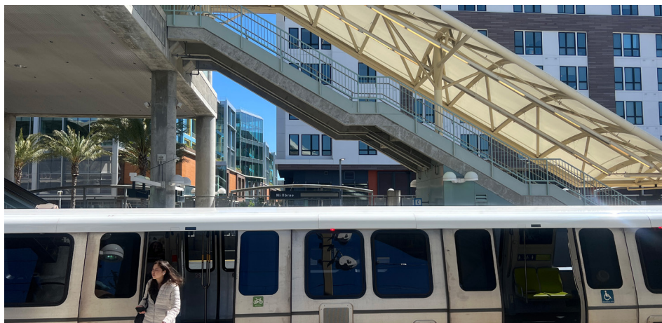
The Gateway at Millbrae, pictured in the background, includes 400 new residential units, including 80 veteran-preferred affordable units; 157,000 square feet of office space; 44,000 square feet of mixed-use retail; and a 164-room hotel.
