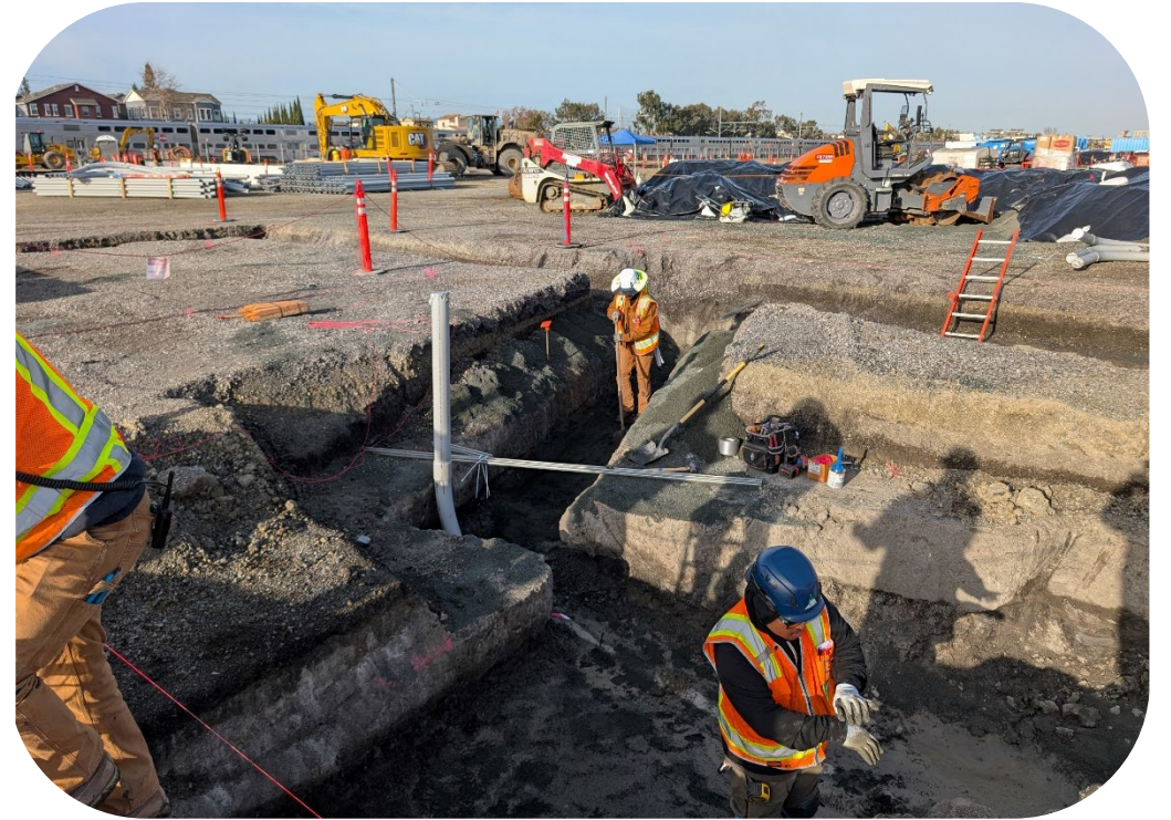
Installing lateral utility connections.
