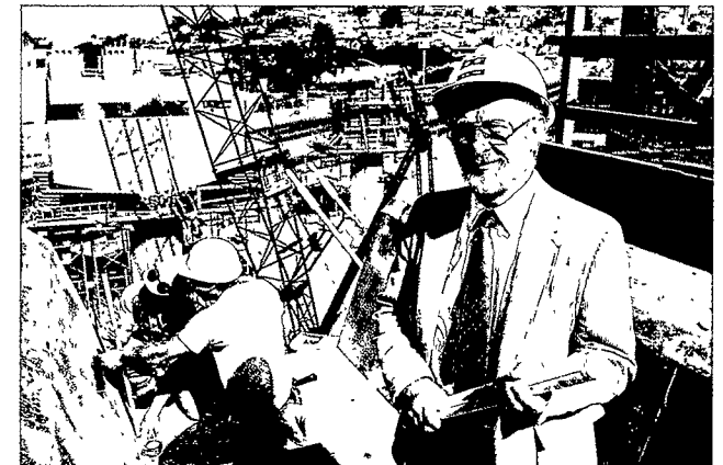
Robert W. Mix, Project Manager of the Daly City Turnback and Storage Yard, completion of which is expected late in 1988
