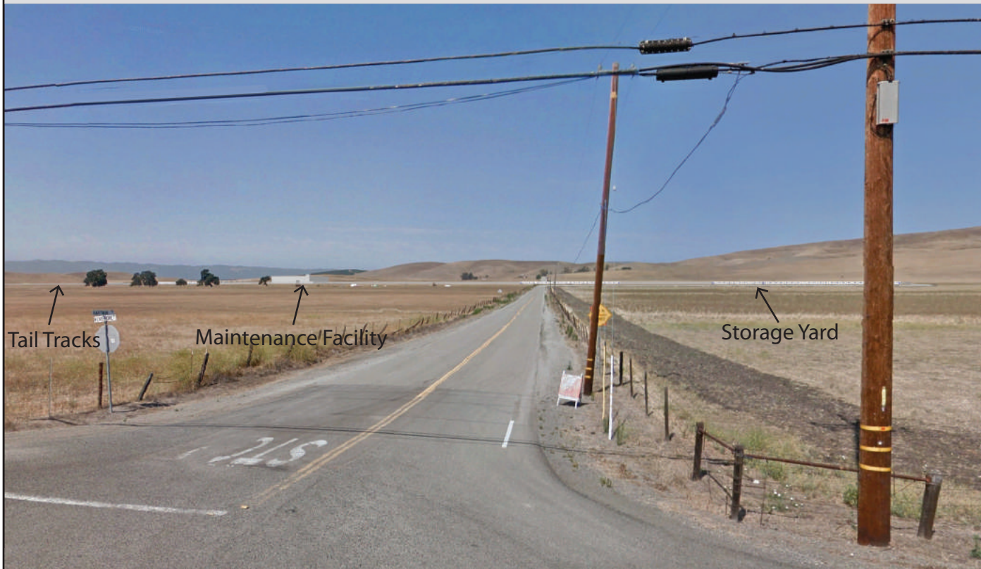
Viewpoint 10: West along Hartman Road at proposed storage and maintenance facility
