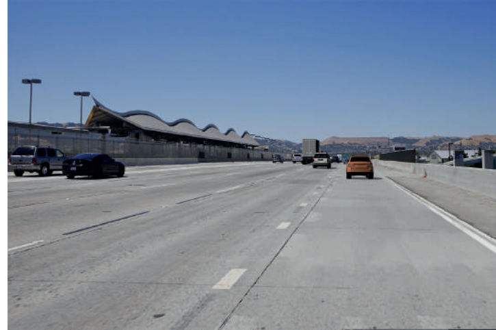
Viewpoint 2: View from I-580 westbound towards the Dublin/Pleasanton Station.
