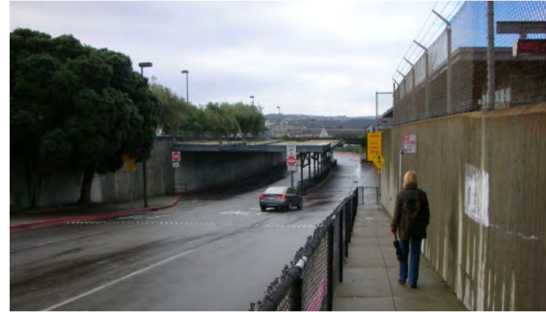
Figure 7-14 East Station Road Security Fencing
