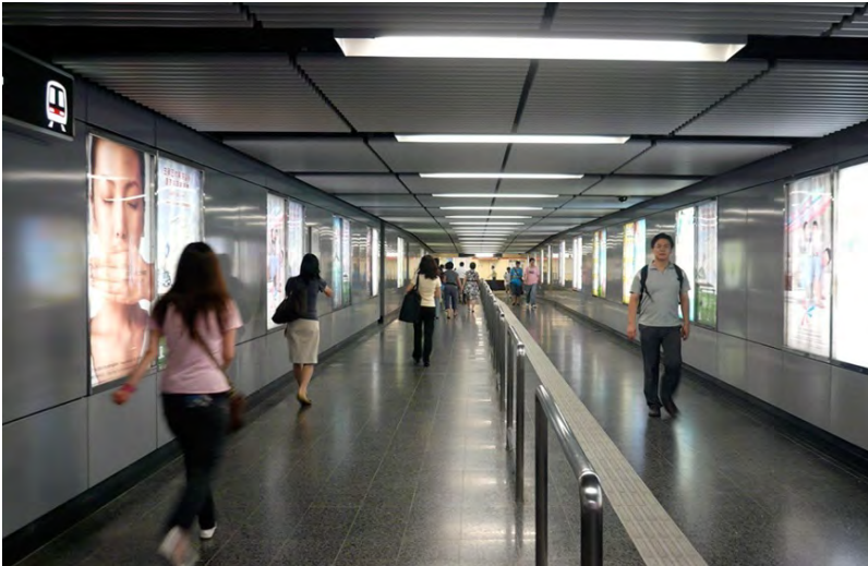
Figure 7-3 Pedestrian Tunnel in Hong Kong
