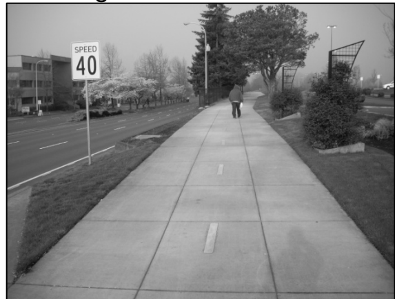
I-205 multi-use path, parallel to SE Sunnyside Rd. near SE 93rd Ave.
