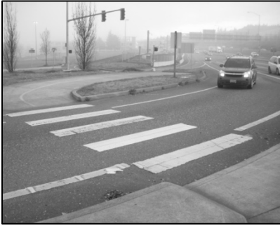
Clackamas County: I-205 multi-use path and I-205 off ramp to SE Sunnyside Rd.
