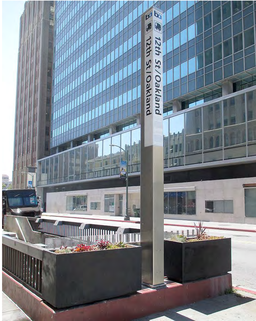
Figure 2.1.1.3: Station identification pylon at underground station entrance
