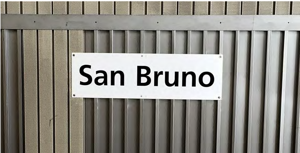
Figure 2.1.2.2: Wall-mounted station identification sign in trackway
