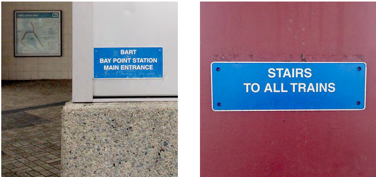
Figure 2.5.1.1: Tactile signs at station entrance and at vertical access
