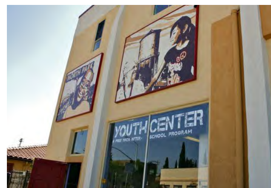
New community facilities should build on existing assets such as the Milton Shoong Chinese Cultural Center (top) and Lincoln Square Park (middle). A youth center (bottom) is proposed.
