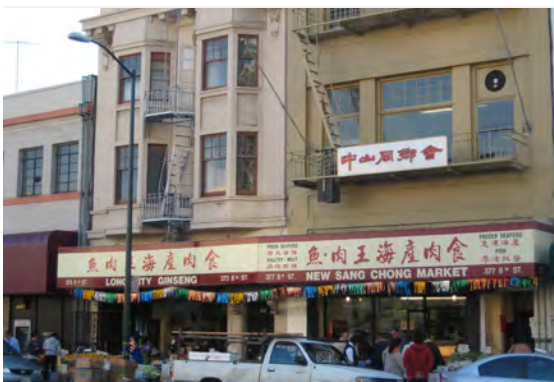
The vision for the Chinatown Commercial Center is to celebrate, strengthen, and enhance this existing community hub and regional destination.
