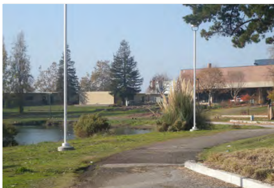
Measure DD-funded improvements currently underway include redesign of the roadway along the Lake’s southern edge (top); building a clear span bridge at 10th Street (middle), and enhancing bicycle and pedestrian access (bottom). These images show conditions before improvements.
