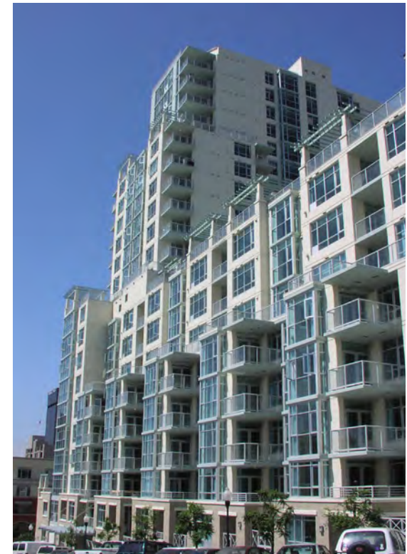
The overall massing, intensity and density of a building could be increased over the base allowance by providing community-identified benefits.
